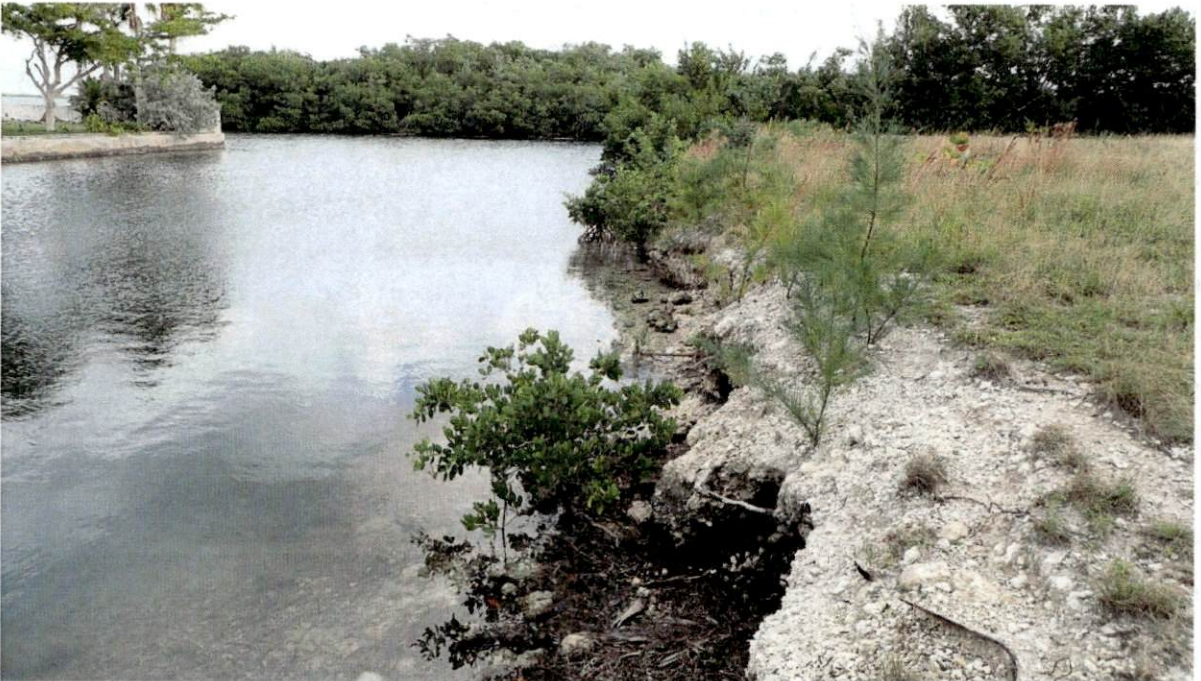
Photo 2. Subject property showing the boat basin with eroding shoreline and the adjacent disturbed upland area.
